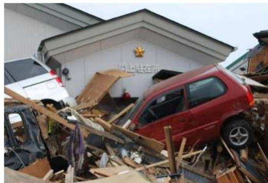
The damaged Yuriage Residential Police Box, Iwanuma Police Station, Miyagi Prefecture
