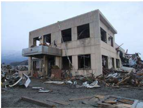
The damaged Takata Police Box, Ofunato Police Station, Iwate Prefecture
