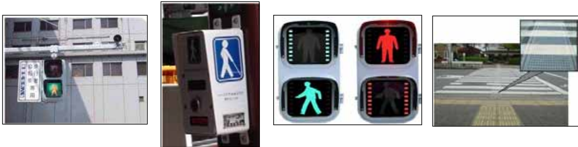
Acoustic traffic signals Traffic signals responding to the elderly Traffic signals for pedestrians to indicate passing time Escort zone
