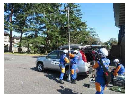
Installing a temporary radio relay station
