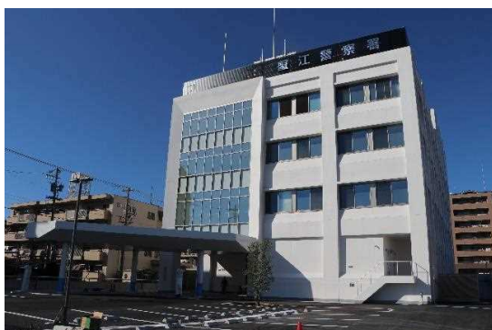
A floor higher than the surrounding streets and office space on the second floor or higher (measures against flooding of the Kanie police station of the Aichi Prefectural Police)
