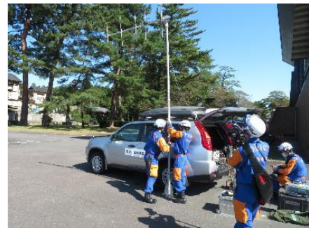
Installing a temporary radio relay station
