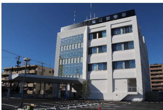
A floor higher than the surrounding streets and office space on the second floor or higher (measures against flooding of the Kanie police station of the Aichi Prefectural Police)
