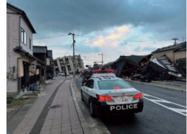
Damage in the affected area
