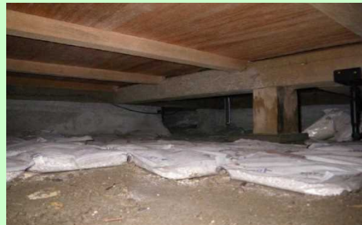
(Mats placed under the floor)
