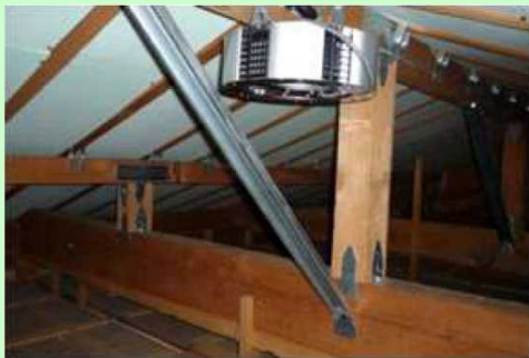
(Unnecessary construction work in the attic implemented by a malicious dealer)
