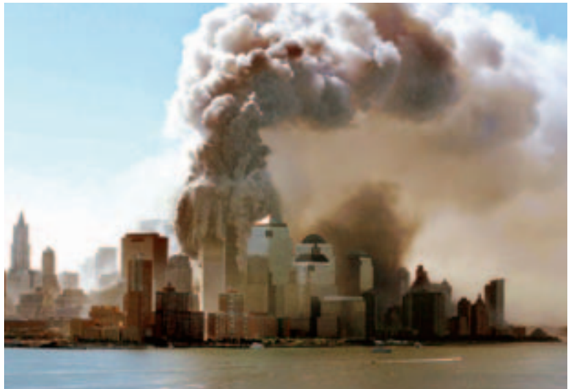
The World Trade Center and other high-rise buildings in Manhattan consumed by flame (September 2001) (Photo: Jiji Press)
