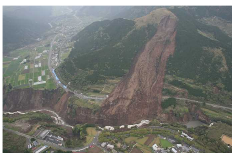
The Aso-ohashi bridge collapses from landslide
